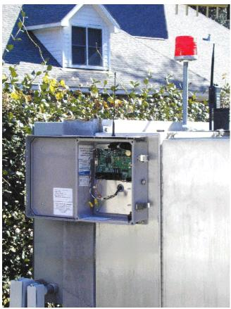
attached to the installation site. The antenna may be remotely mounted up to 50 feet away from the RTU. Call MISSION for extension cables. **Do NOT cut and extend the antenna cable your self!** Remember to seal/plug the antenna's mounting hole on the top of the Model 100 enclosure.
