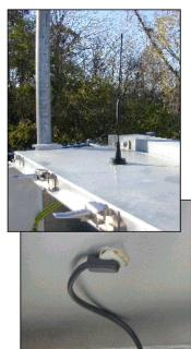
The antenna cable (coax) runs through the pump station enclosure into the Model 100 enclosure which is mounted on the side of the pump station.
