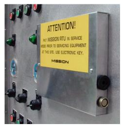
same conduit as the input wires but longer runs could cause problems. Try and mount the supplied AC transformer outside the MISSION enclosure in the control panel near the 120VAC source. This way only low voltage AC is fed inside the MISSION enclosure. Sometimes this is not possible and the transformer must be mounted inside the MISSION enclosure. This is acceptable, but severe voltage spikes could now be introduced inside the enclosure.
