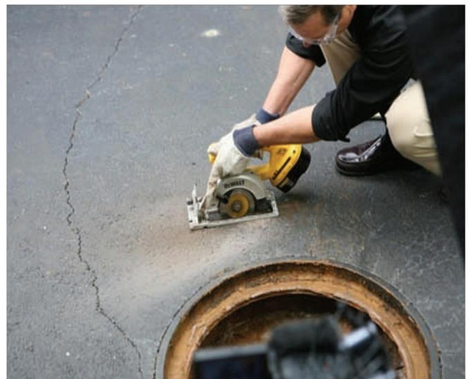
Clean out any loose material from the slit to prevent damage to the antenna or cable. You may want to use the small drill bit to root out the slit of debris or make wider if necessary. Feed the connector end of the antenna cable into the hole and through the sewer vault. Pull the cable through so that the Black antenna elements sit down in the 12” slit in the road and below the road surface.
