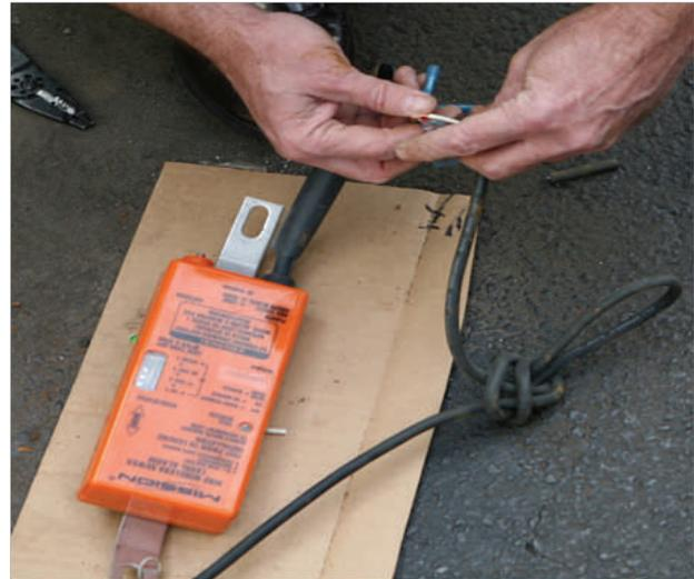
Make sure the heat shrink tubing is on the M-80 wire harness before making connections as this will be placed over the connections once the wires are terminated and the blue connectors are heated.
