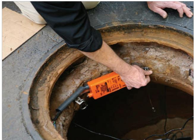
Tighten the nut clockwise onto the bolt. This will expand the masonry bolt to secure it into the hole. Next, loosen the nut and remove the nut and washer from the bolt. Slip the end of the M-80 stainless steel strap over the mounting bolt. Place a washer and nut on each bolt and securely tighten.
