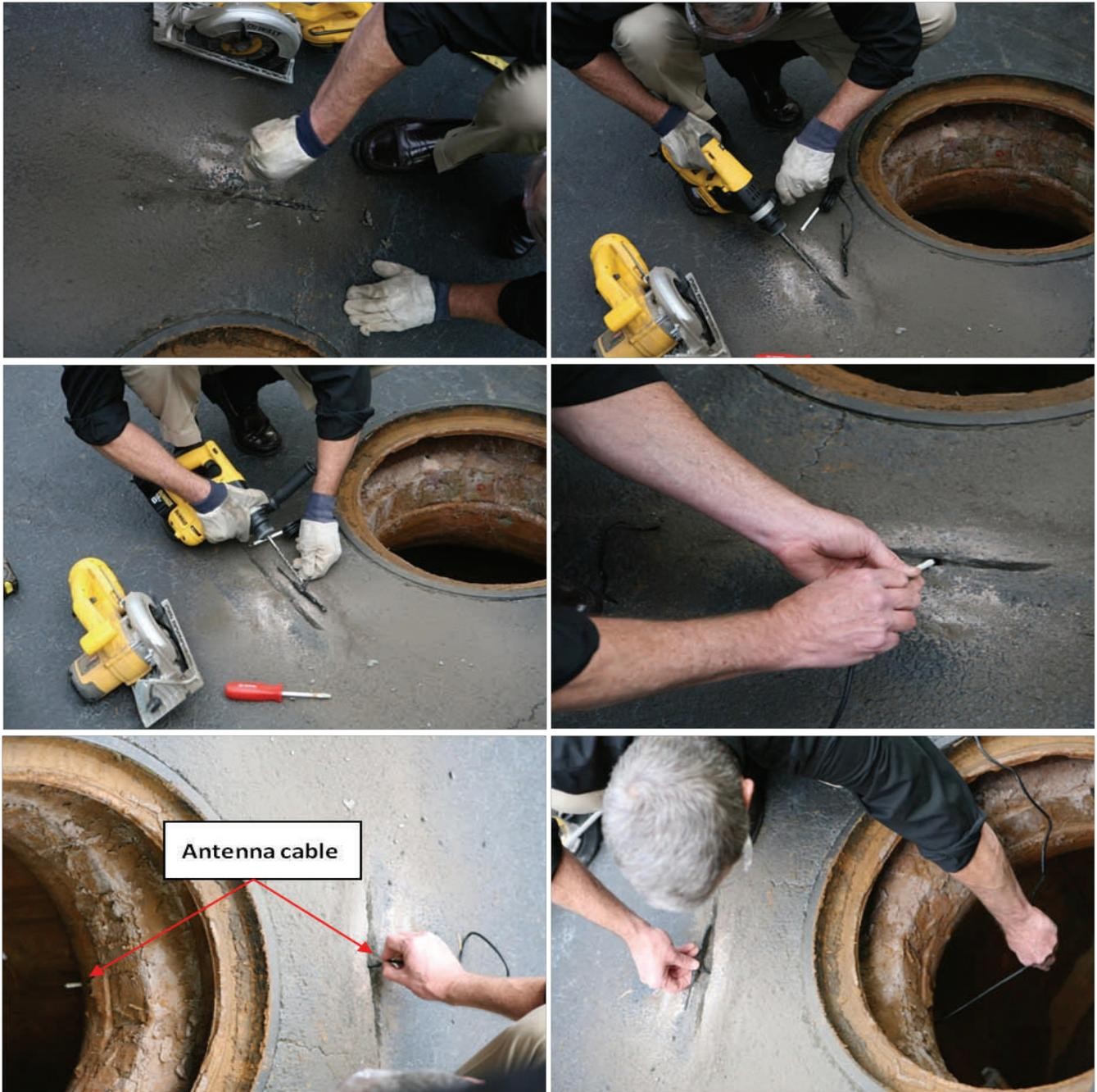
Once the antenna is seated correctly, apply the road tar sealant (included) on top of the antenna and slit. After the asphalt sealant is injected into the groove, use the included plastic knife to work the sealant into the groove and to smooth its surface.
