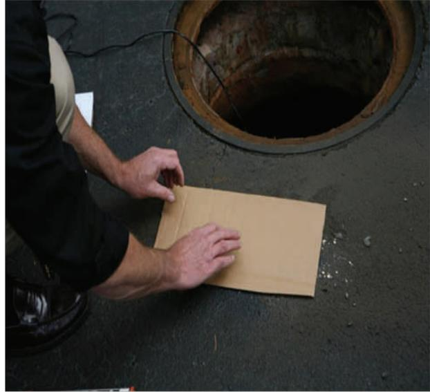
The asphalt sealant placed into the antenna groove cut into the road or sidewalk is sticky for about four hours. The oatmeal/cornmeal speeds the drying of the sealant and prevents the tacky sealant from being drawn out of the groove by foot or road traffic while it is drying!
